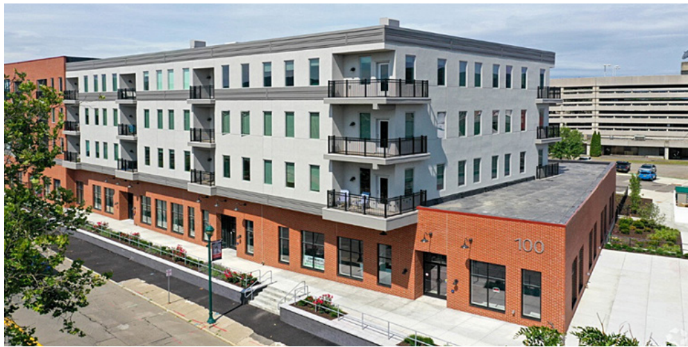
100 W. Water Street Apartments, Elmira
