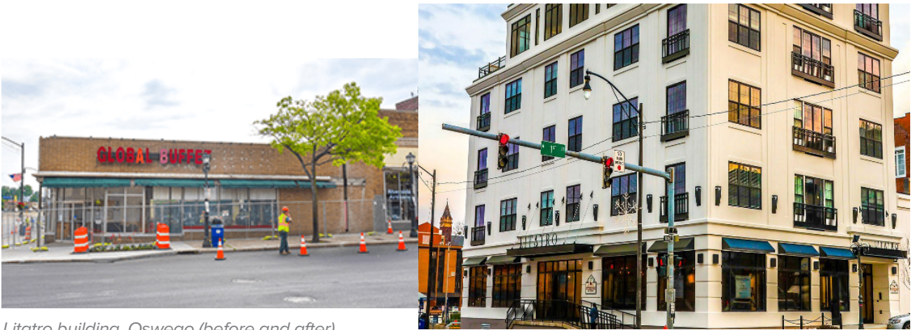
Litatro building, Oswego (before and after)
