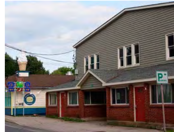
The Orvette Building has been rehabilitated into workforce housing and has a waiting list for tenants.
